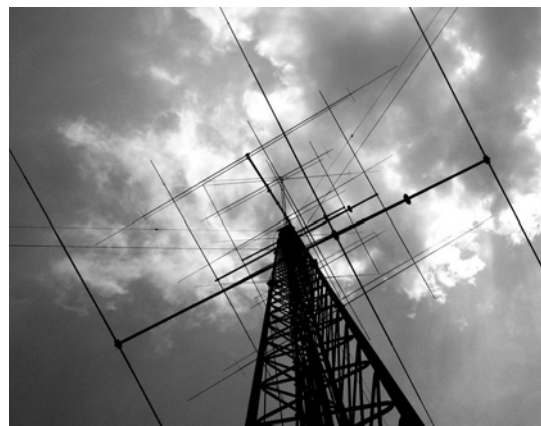
One of the towers at W1AW, shown below.
